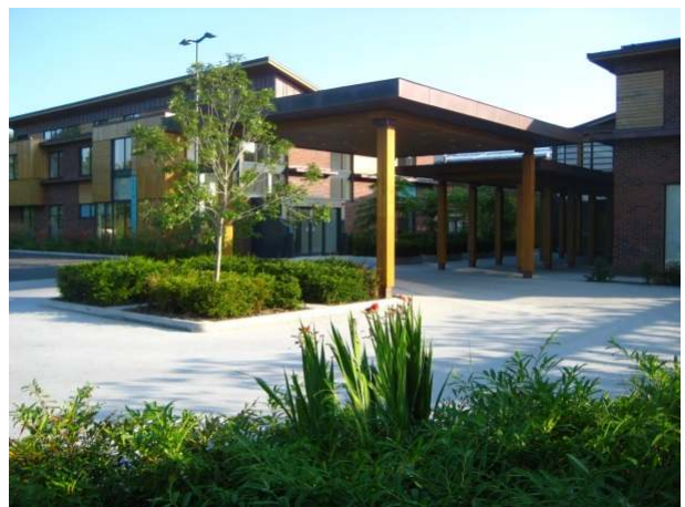
ST. FRANCIS HOSPICE BLANCHARDSTOWN
